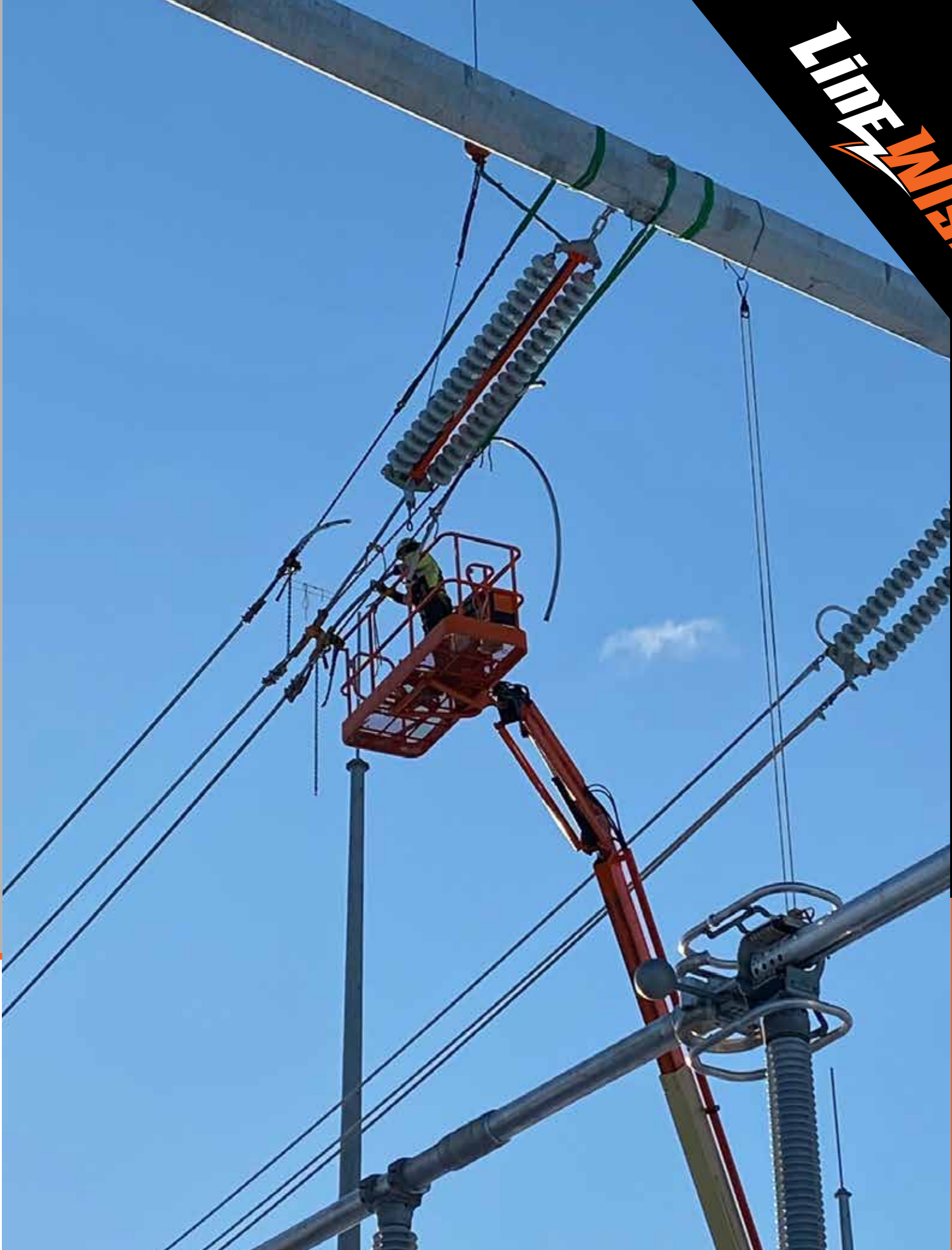
Quad/Tri Bundle Insulator Spreader
