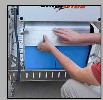
Battery removal is quick and easy. Remove cover, disconnect 2 cables per battery and remove battery.
