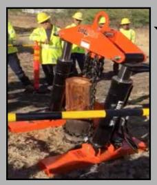
Stub Puller option allows removal of poles that have been cut off above ground level, but at a height too low to pull out with the standard Pole Puller. Pole Puller successfully removes poles that are foamed in rocky soil!
